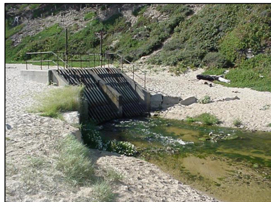
Figure 4:6 - The mine adit that now prevents water levels being too high in the Loe Pool and in turn helps reducing flooding along the River Cober. (Source: Helston History, 1999.)
