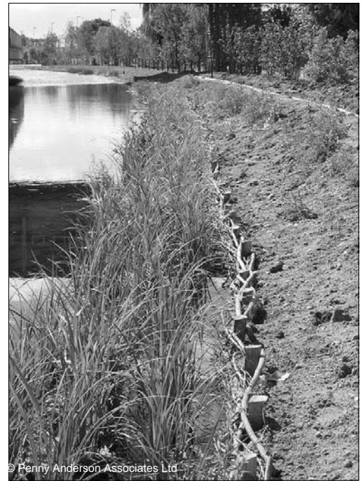
← Newly created berm → willow / hazel spilling to retain stability of bank → bank cut in sub-soil with appropriate seed mix
