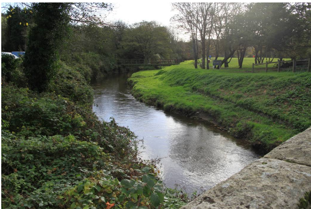
River Cober immediately downstream of Zacharys Bridge – Two-stage flood channel constructed in 1988 as part of Helston flood defence works
