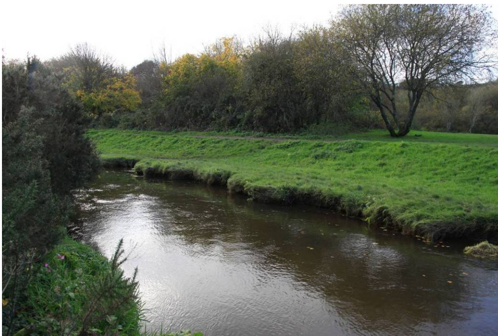
River Cober downstream of Zacharys Bridge - Two stage flood channel constructed in 1988 as part of Helston flood defence works
